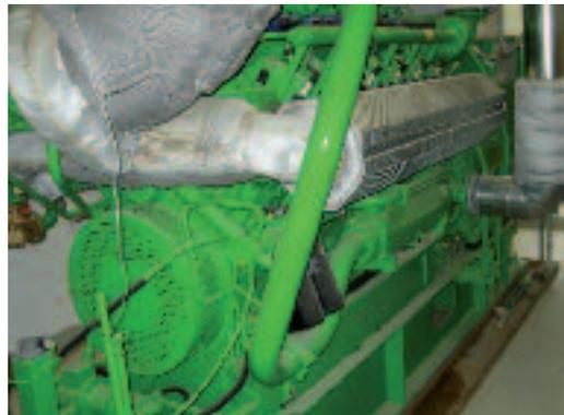
**CHP Biogas Engine**
